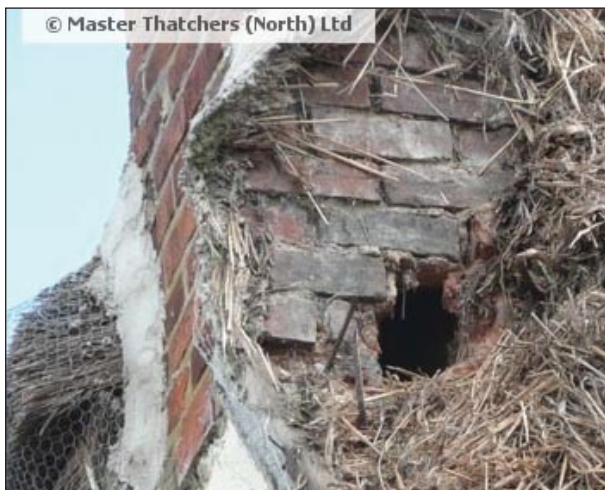
Above, thatch removed from around the chimney.
