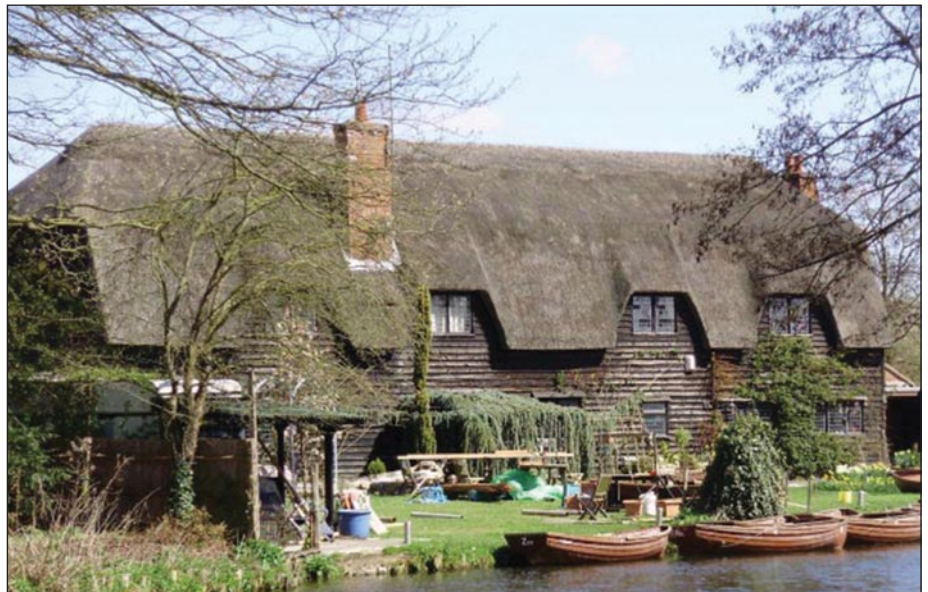
Above, a detailed understanding of the Building Regulations is required.
